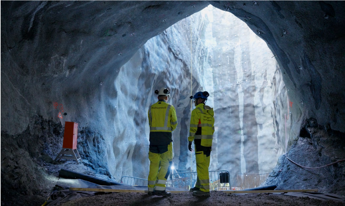
Construction of Fornebubanen | Photo: Sigbjørn Holthe/Multiconsult Norge
