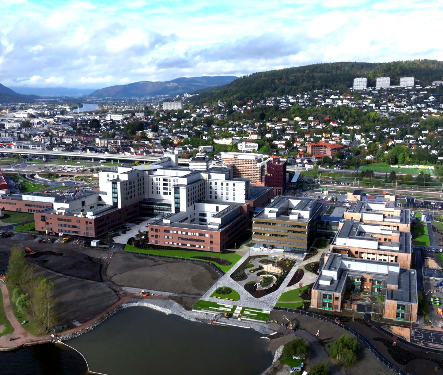
The new hospital in Drammen | Photo: Multiconsult Norge
