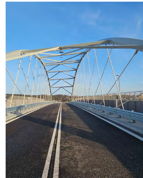
Viaduct, Gdynia | Photo: Multiconsult.
