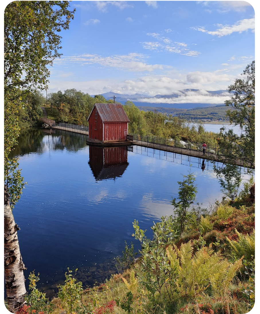
Slettaelva dam | Photo: Multiconsult
