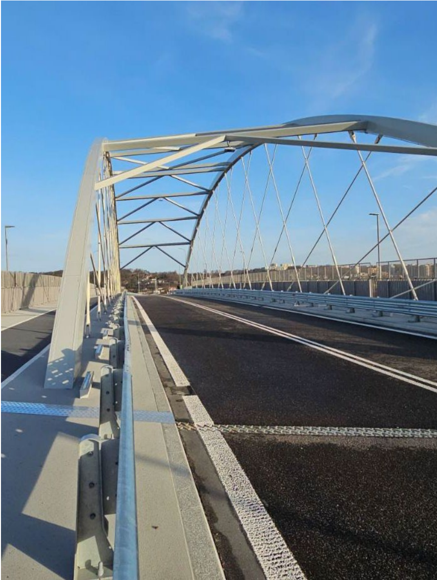
Viaduct Gdynia, Poland | Photo: Multiconsult
