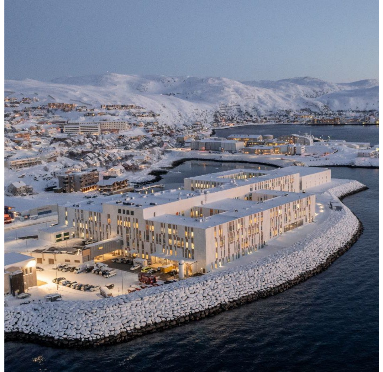
New Hammerfest hospital | Photo: Tor Even Mathisen, Finnmarkssykehuset
