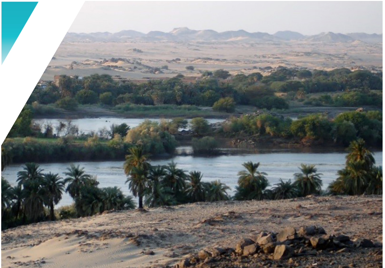
The Dal Hydropower Project is located on the Great Nile in Northern Sudan
