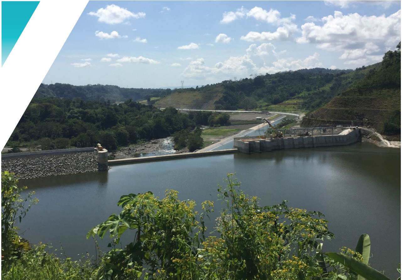
Bajo Frío reservoir and headrace canal | Photo: Jørn Stave, Multiconsult
