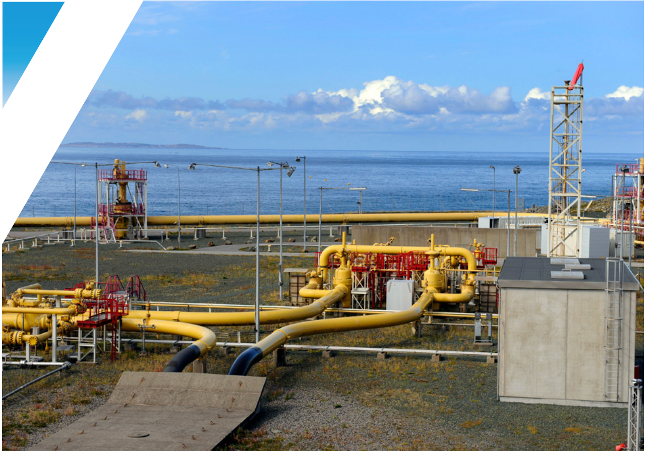
Kalstø Landfall | Photo: GASSCO
